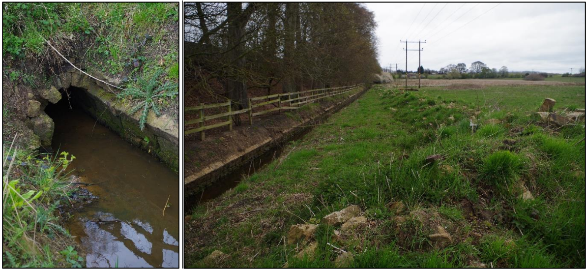
Plate 4. Left: a piece of intact culvert at Myers Flatt and right: the exposed stone lined ditch without its capping and rubble alongside which includes reused stone sleepers. The 1825 embankment runs along to the left.
