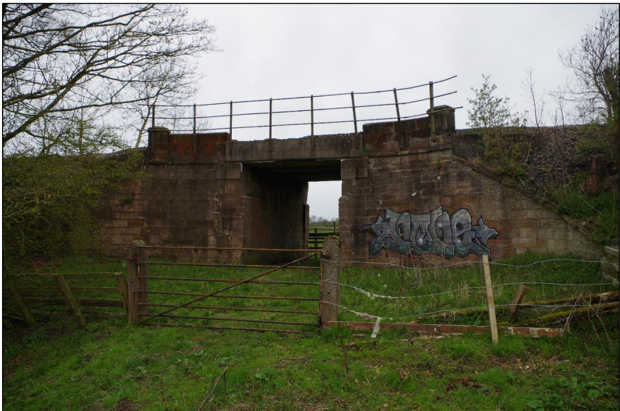
Plate 6. Accommodation bridge at Myers Flatt
