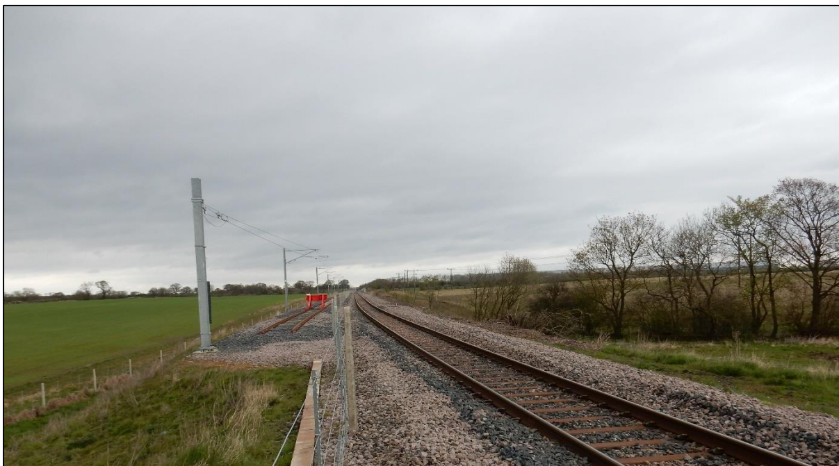
Plate 1. Additional track bed recently built for Hitachi on the left
