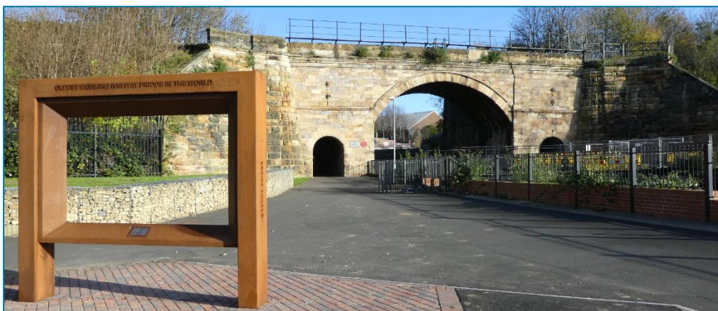
[7] Skerne Bridge (photo © Gaby Rose, November 2024): Railway bridge designed in a classical style by Ignatius Bonomi for the S&DR, 1825; subsequently altered/strengthened. It is the only architect-designed bridge of the S&DR 58 and featured on the company's headed paper. It is now the world's oldest railway bridge still in use, as stated on the recently installed metal artwork in the foreground. Also note the vegetation growth on the bridge, which is a concern for its structural integrity (see section 4.2). Whilst the galvanised lighting column in front of the bridge detracts from the view, the recent works to the river-side railings by Northern Gas Networks have improved the setting of the bridge 59 .
