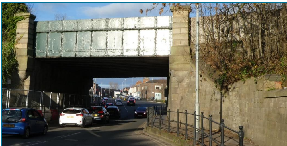
[6] Railway Viaduct (photo © Gaby Rose, November 2023): Plans to build the bridge had begun in the 1840s. It was finally built in 1856, altered/rebuilt in 1876, and the road level further dropped after 1949 to allow for double-decker busses 107 . An early photograph shows a plaque with the date MDCCCLVI on the side. Altered prior to 1935.
