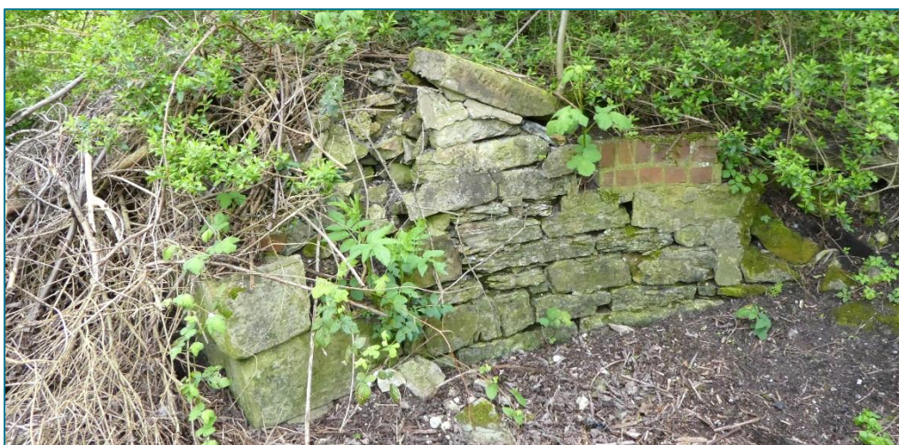
Top: Remains of [G] Enclosed Railway Corridor in Pease brick laid in the English Garden Wall bond to the north of the former Gas Works and windmill sites; note the 'zigzag' line of wall (Photo © Gaby Rose, March 2024). Middle: Remains of later, southern coal drop walling of the [D] Coal Depot built in stone; the brick walling on top was added when the depot was no longer in use. The wall now forms the boundary to the carpark of the former [E] Fighting Cocks Inn. Bottom: This feature, judging from its position near the [A] Crane Base and Platform just outside this view on the right/north (see below), seems to be related to the ramp carrying the siding track to the coal cells. (Photos © Gaby Rose, April 2024)
